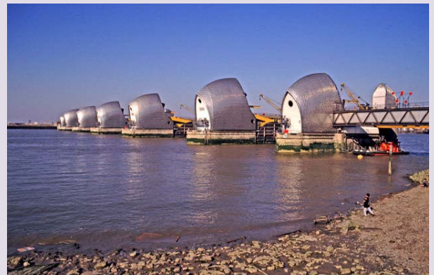
Thames Flood Barrier – built to prevent the floodplain and eastern Greater London from being flooded by high tides and storm surges. Photo credit: Wikimedia Commons.
