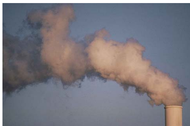
Air Pollution: Smoke rising from a plant tower. Photo credit: Wikimedia Commons.
