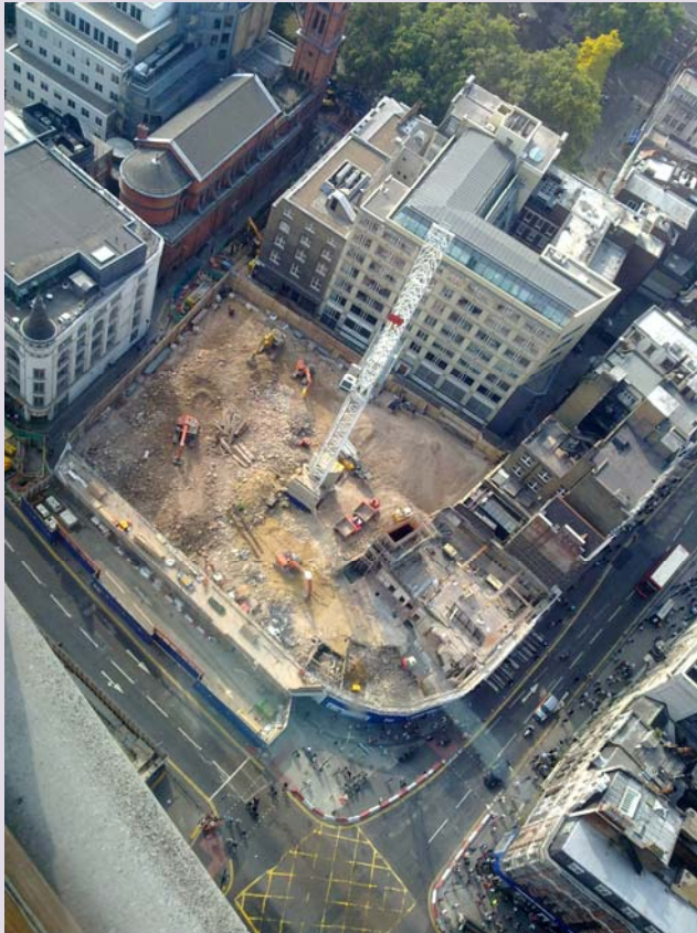
The Tottenham Court Road Crossrail construction site. Photo credit: Wikimedia Commons.
