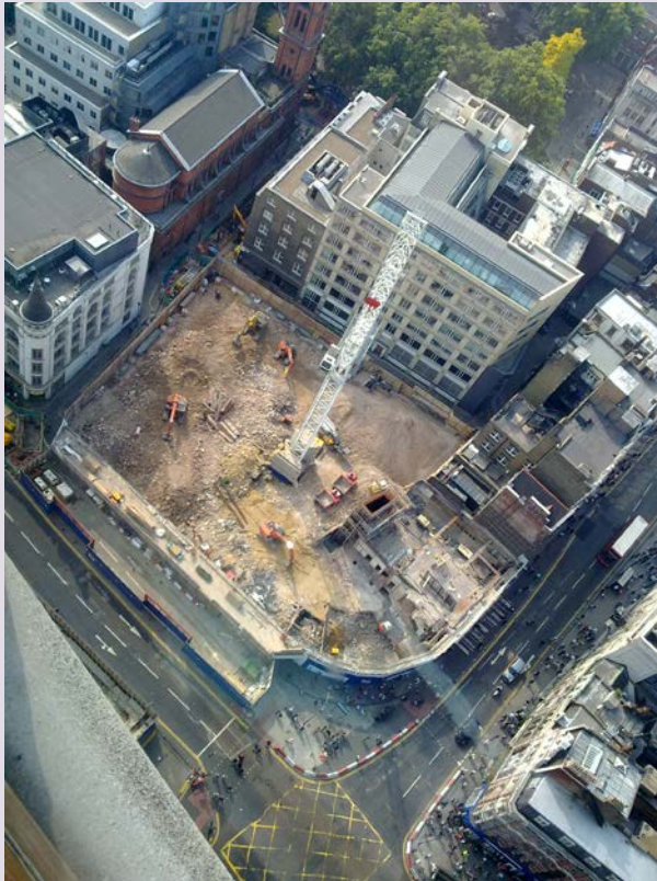
The Tottenham Court Road Crossrail construction site.
